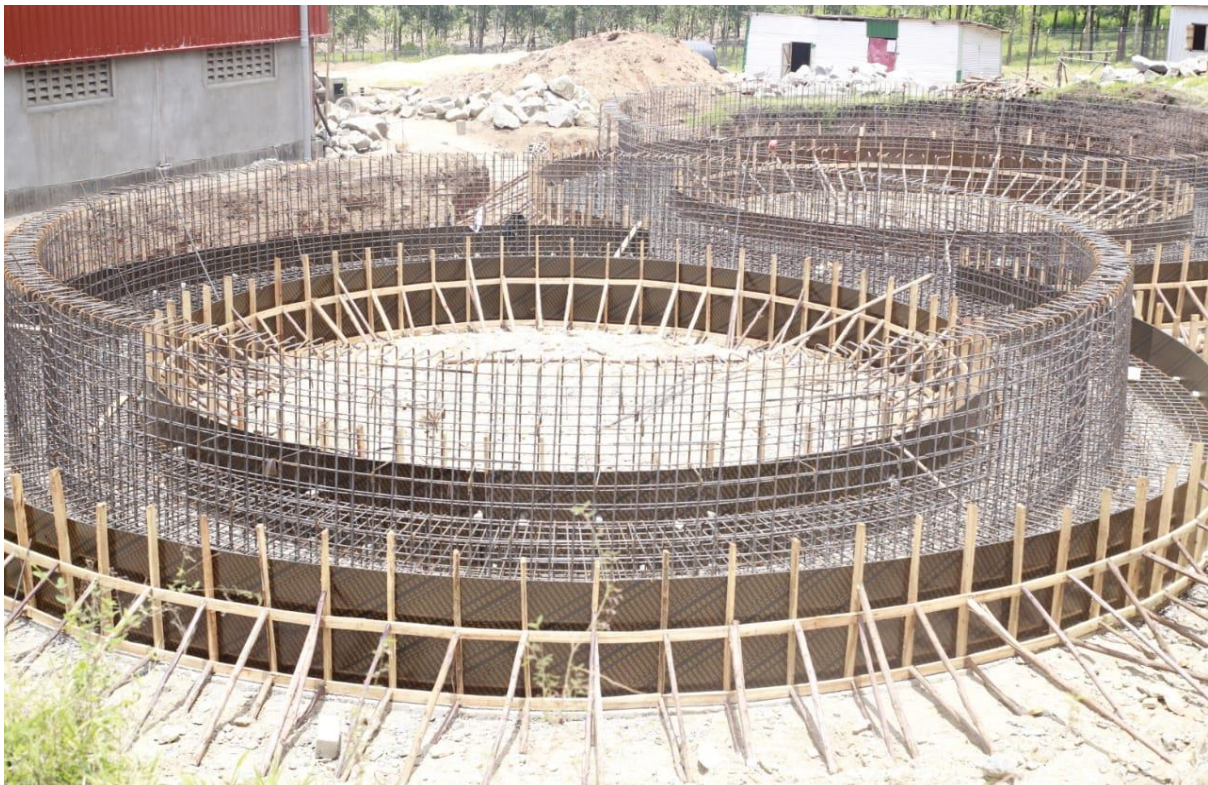
Figure 21: A 3,000MT twin Silo base under construction at U.G Prisons Farm Ruimi.
